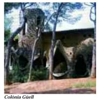
Bellver (interesting brickwork decoration). The most outstanding building is the crypt (1898-1915) of the unfinished church, commissioned by Güell to Gaudí. One of Gaudí's most frequently studied works on account of the structural innovations -columns slanted according to the weight they have to bear, parabolic and hyperbolic roofs-, the superb use of materials -basalt stone and brick studded with polychrome mosaics and stained glass windows- and the spaciousness of the inside and the porch. The
