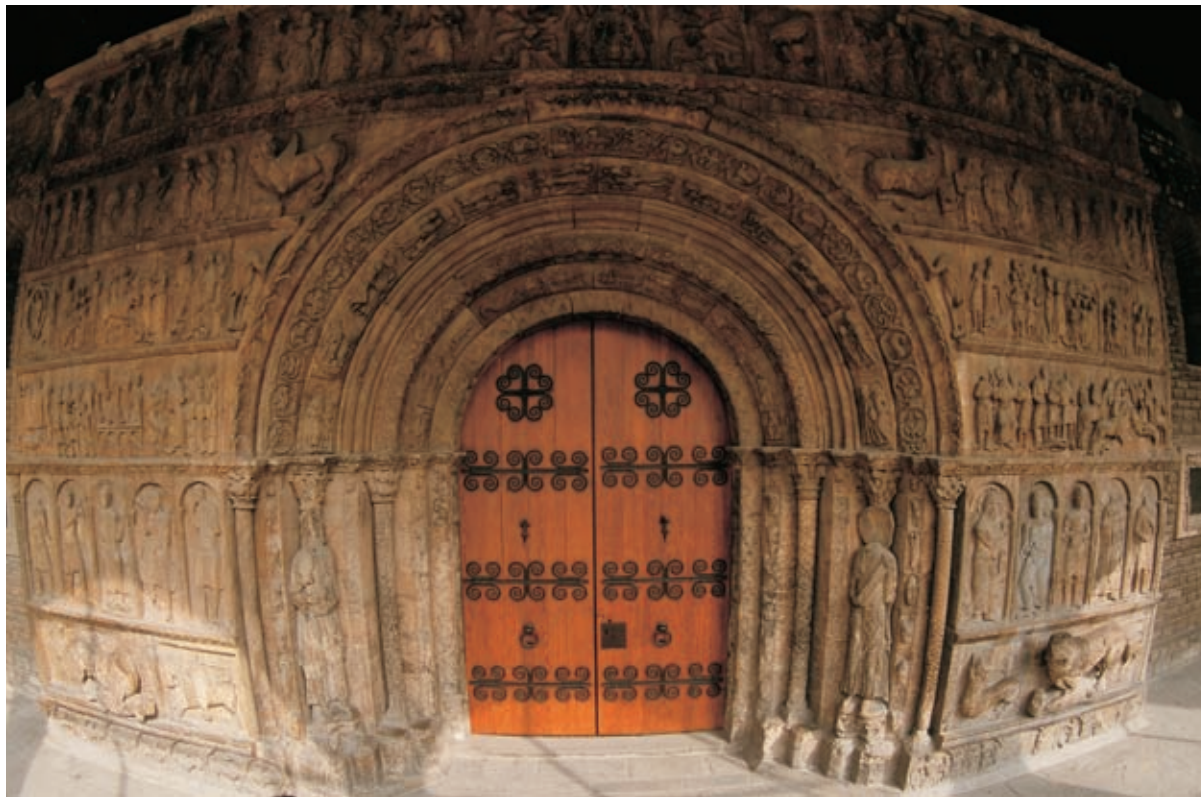
Ripoll. Doorway, Santa Maria
